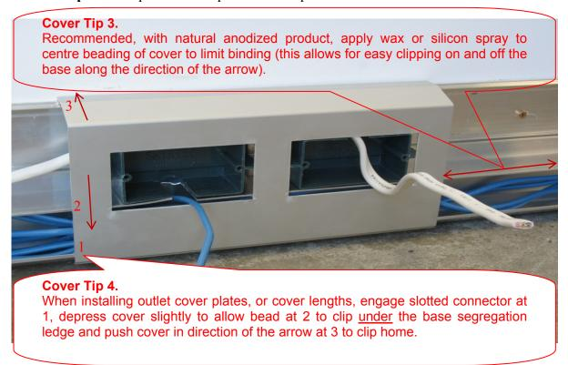
Once outlet kits are in position the installation may be covered up through the installation of covers, corners and ends.
