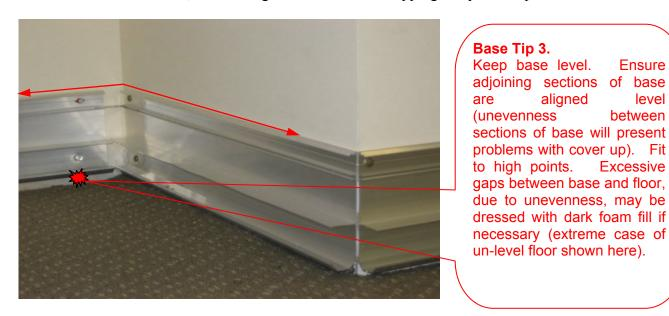
• Do not stress base into the wall, pack out if necessary and fasten into high points.
