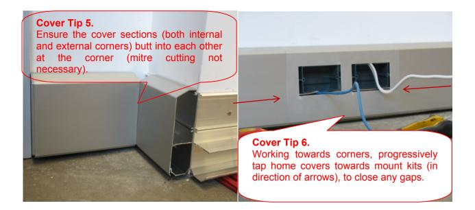
• Clip home corners. Engage the top tab into the back of the cover and press home the bottom lugs (listen for a definite 'click' home on both sides of the corner).
