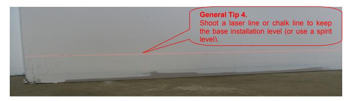
• Use appropriate tools and fasteners for attaching the base section. Generally fasteners are to be used along the base, top and bottom, with centers no greater than 800mm (into studs where applicable). Liquid nails may also be used as an addition to other fasteners.
